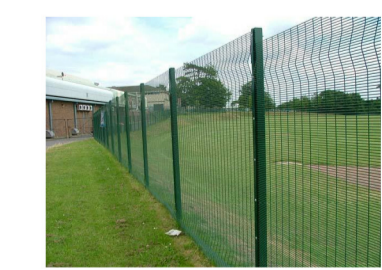
Example of mesh welded wire boundary fence
